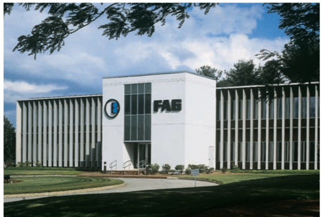
Barden Super Precision Bearing plant in Danbury, Connecticut, U.S.A.
